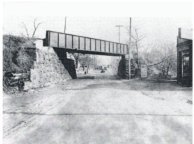
Jericho Turnpike looking east from Little Neck Parkway before the Creedmoor freight spur trestle was replaced with a wider one in 1931. Newer trestle is now also gone.
