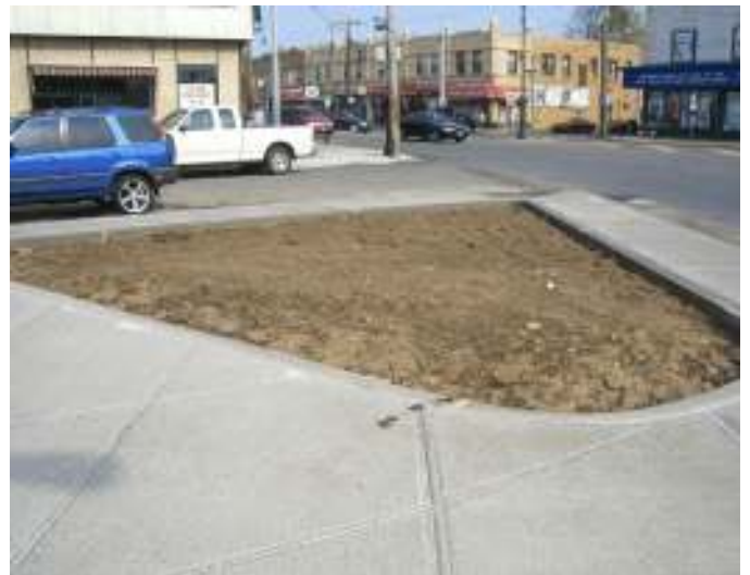
City DOT reconstructs corner of 245 th Street and Braddock Avenue.
