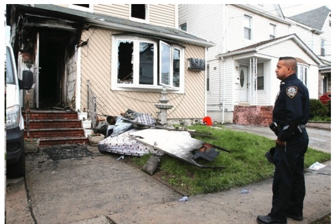
Police officer surveys damage to Queens Village house.
